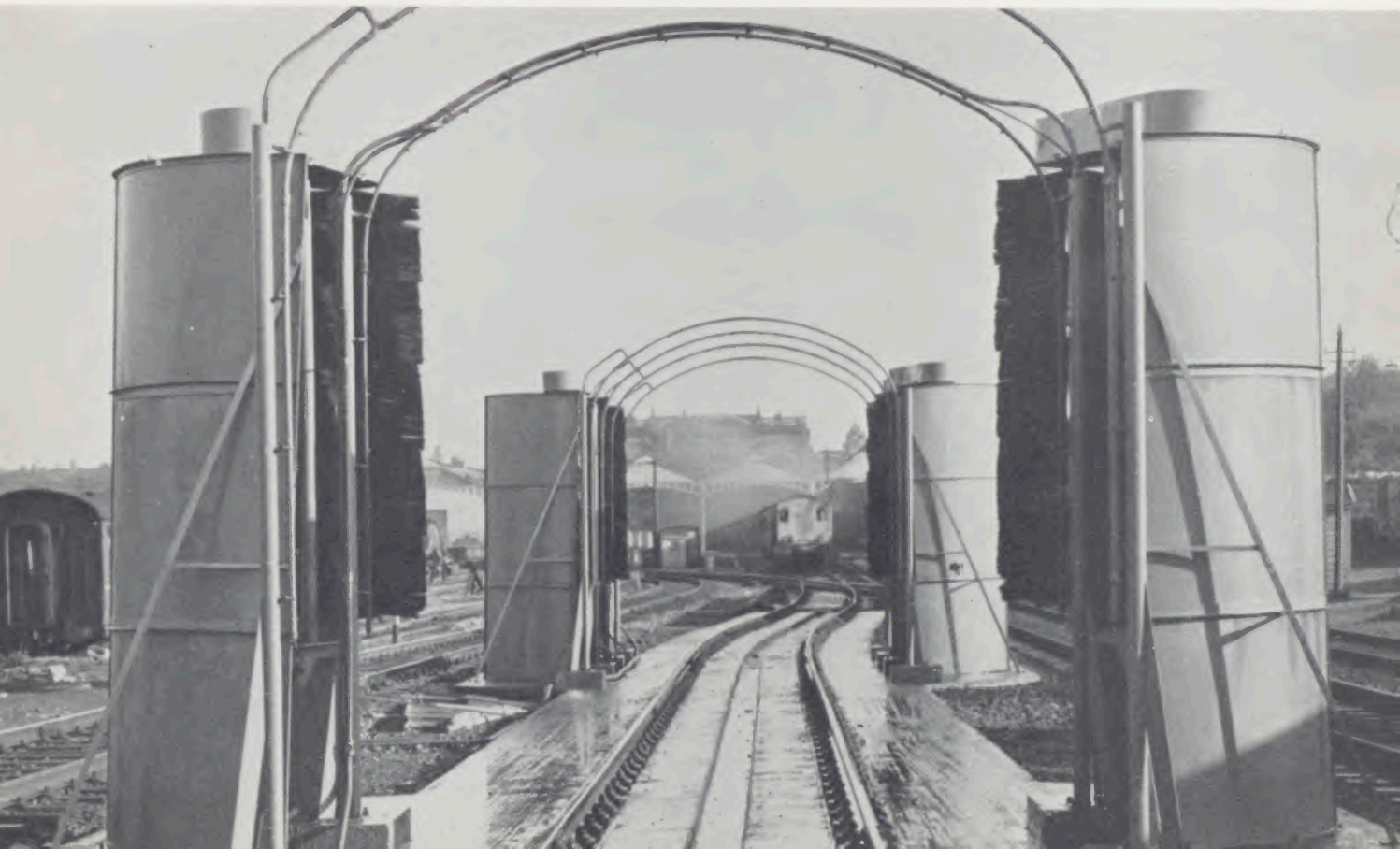
Train washing plant at Kingsbridge.
