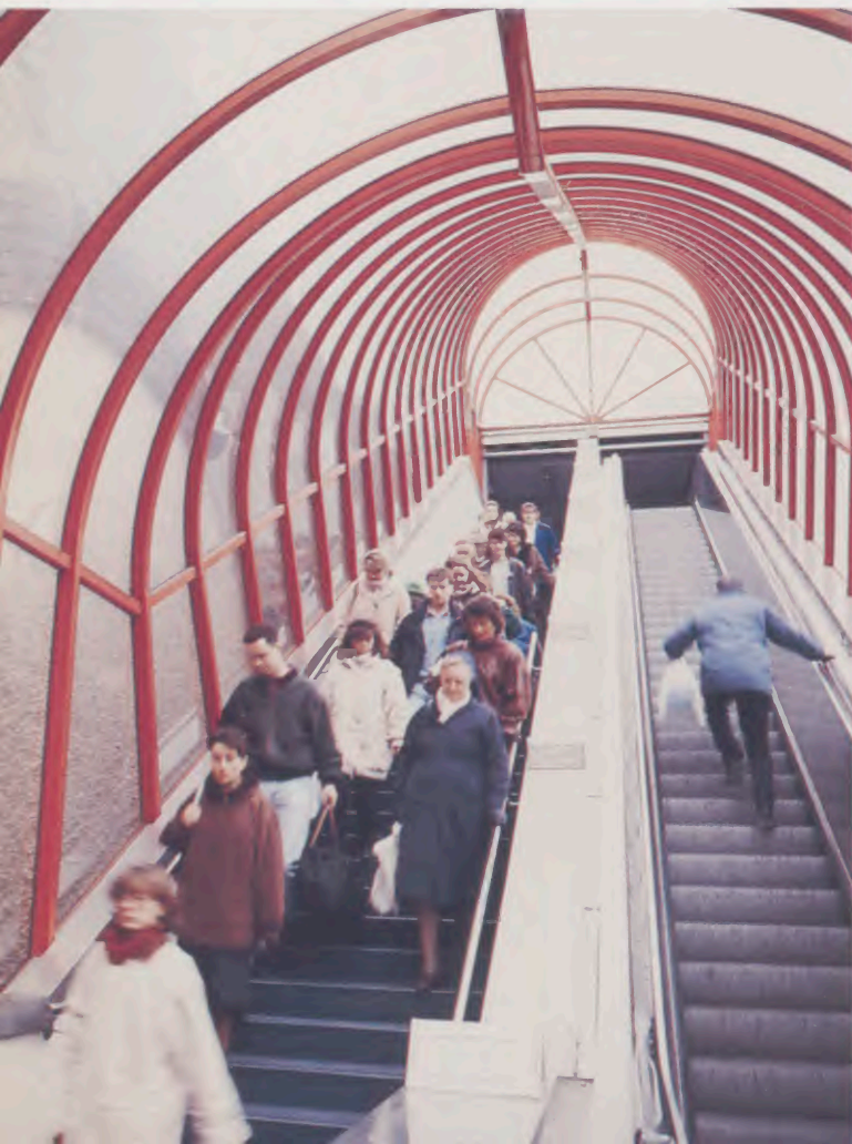
Tara Street Station, which underwent a major refurbishment programme
