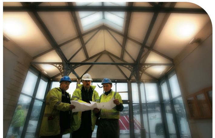
Renovation work at one of our bus stations
