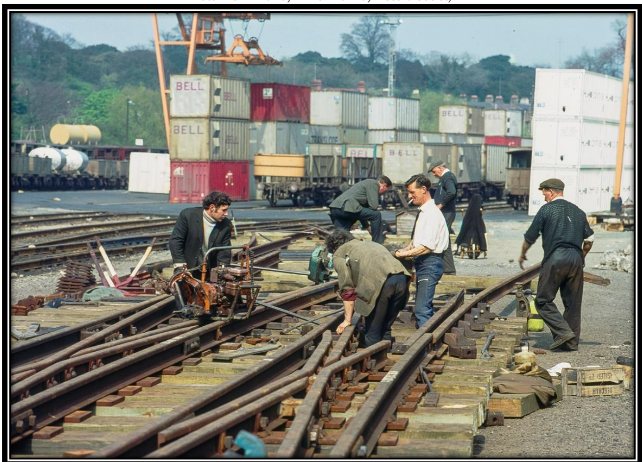
PWDept_1970s_Heuston_Jul_1974_IrishRailwaySociety.jpg Permanent Way Dept. assembling tracks and points at the new freight container yard at Heuston Station, July 1974. Photo: Irish Railway Record Society.
