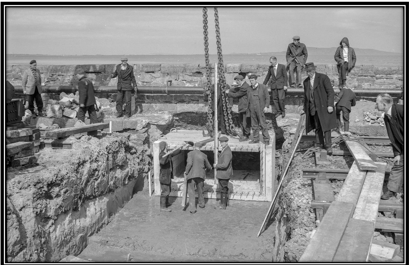
PWDept_1960s_Booterstown_Apr_1968_IrishRailwaySociety.jpg Permanent Way Dept. installing new culvert below the line near Booterstown, April 1968. Photo: Kevin Murray – Irish Railway Record Society.
